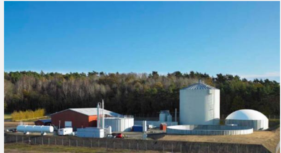
Figure 15 : Installation de Falkenberg (ENEA Consulting, 2010)
